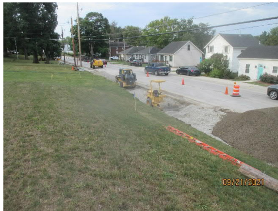
View of water main construction area looking south.
