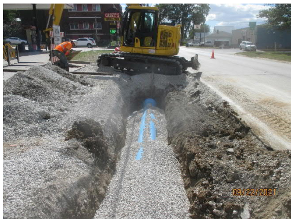
View of 15" PVC storm sewer and initial stone backfill.
