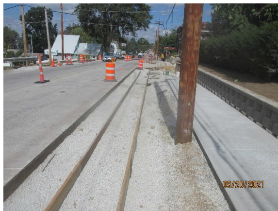
View of curb and gutter forms looking north along Hwy 84.
