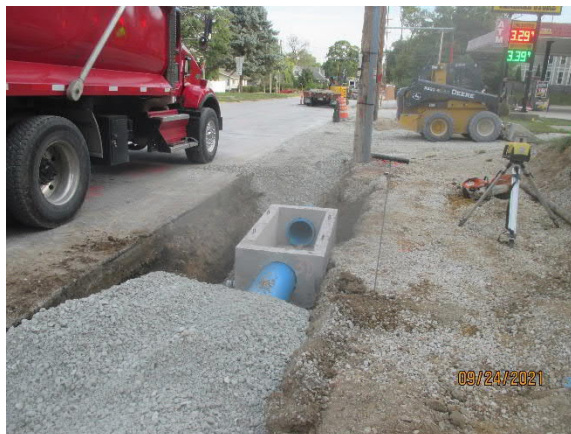
View of PVC storm sewer and inlet special along Hwy 84.
