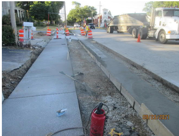
View of curb and gutter and 5" PCC Sidewalk looking south.
