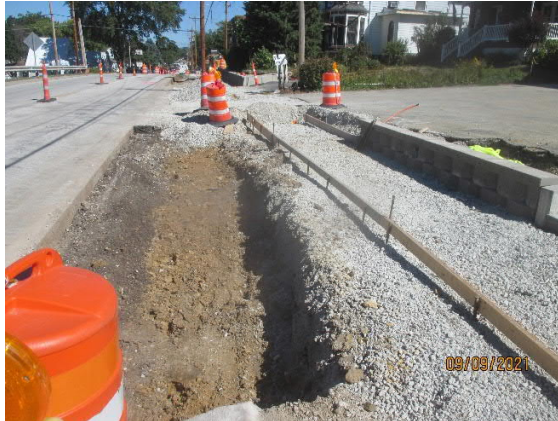
View of curb core out and PCC Sidewalk forms looking north.
