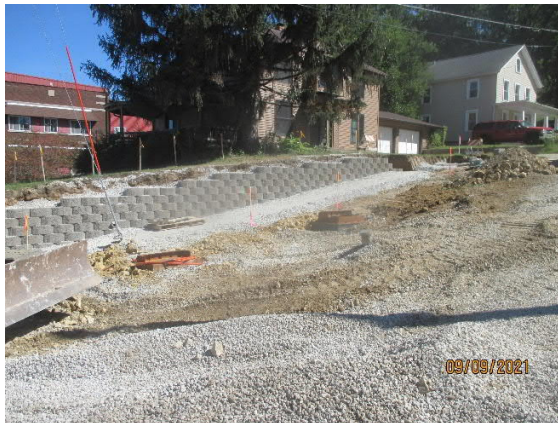
View of installed block wall section north side of Walnut Street.
