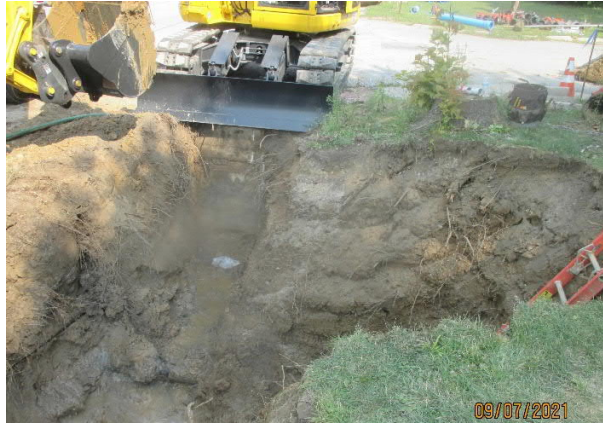
View of existing 6" DIP water main near Taylor Drive.
